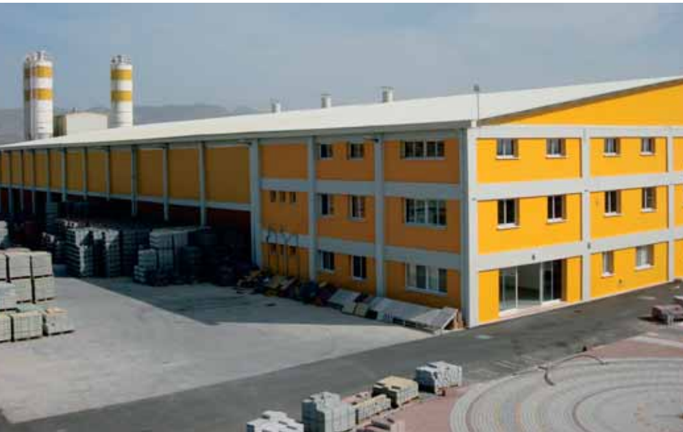
View of the Gürdag production facilities
